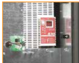
solid-state variable speed control
